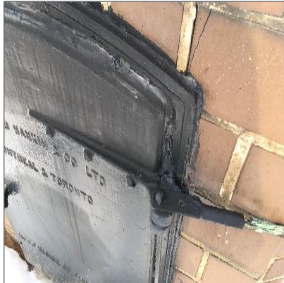
Asbestos-containing black caulking around the exterior frame of the chimney door – Exterior of Boiler Room (samples S064A-C).
