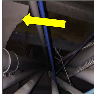
Transite board above slanted lay-in ceiling tiles, north end of Basement Main Corridor.
