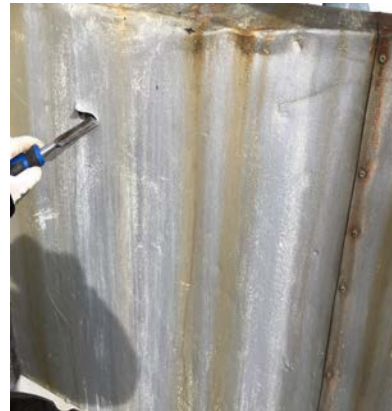
Asbestos-containing preformed block and parging cement insulation below metal jacketing on boiler breeching, Exterior of Basement Boiler Room to Chimney.
