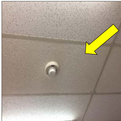
Asbestos-containing 24" x 48" lay-in ceiling tiles, pinhole and texture pattern, Basement ECG Department.
