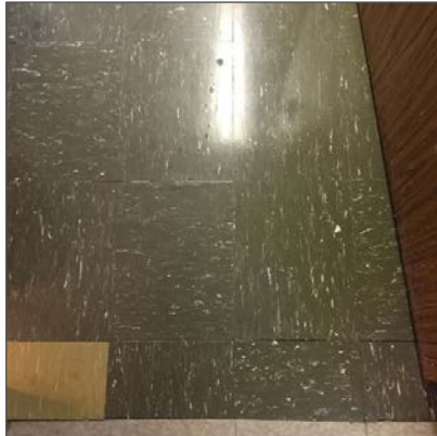
Photo 1 - Asbestos-containing 12" x 12" vinyl floor tiles, green with white streaks and yellow with white streaks, Basement Office #1.
