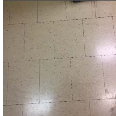
Photo 2 - Asbestos-containing 12" x 12" vinyl floor tiles, beige with thin brown streaks, Basement Locker Room at ER Wing.
