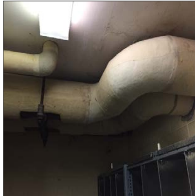
Asbestos-containing parging cement on pipe fittings, Basement File Storage Room.
