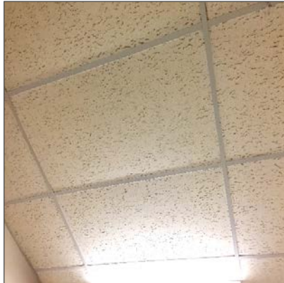
Photo 1 – Asbestos-containing 24" x 48" lay-in ceiling tiles, length-wise fissure and small pinholes, Ground Floor Corridor.
