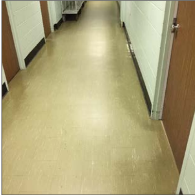
Photo 1 – Asbestos-containing 12" x 12" vinyl floor tiles, yellow with white streaks, Basement Main Corridor.
