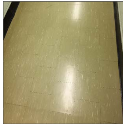
Photo 2 – Asbestos-containing 12" x 12" vinyl floor tiles, dark green with white streaks, Basement Main Corridor.
