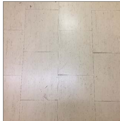
Photo 4 – Asbestos-containing 12" x 12" vinyl floor tiles, beige with thin brown streaks, Basement Locker Room at ER Wing.
