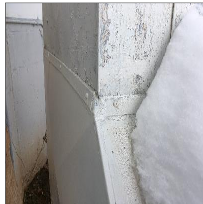
Non-asbestos white caulking at the pleats on the exterior duct work for the HVAC unit – Exterior Boiler Room (samples S068A-C).
