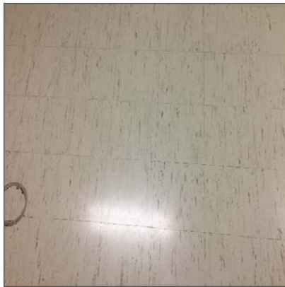
Photo 1 – Asbestos-containing 9" x 9" vinyl floor tiles and mastic, beige with grey streaks, Basement Main Corridor.
