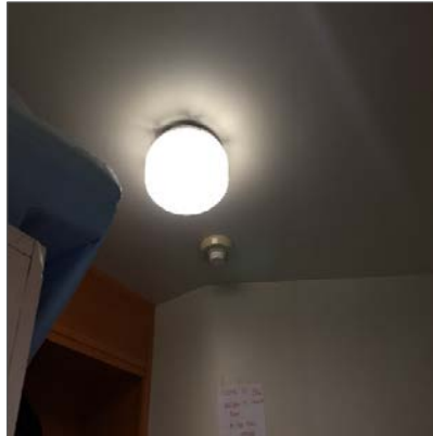
Asbestos-containing paper heat shield in incandescent light fixture, First Floor Storage Closet.
