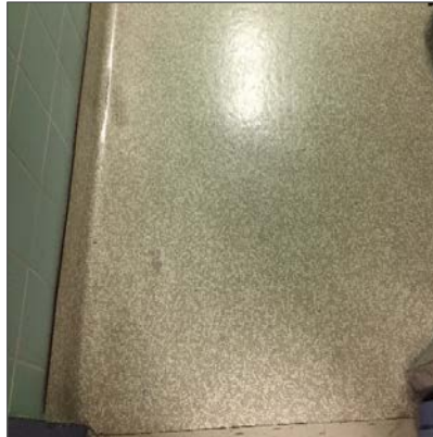
Asbestos-containing vinyl sheet flooring, brown with white squares, Ground Floor Barrier-Free Shower Room.
