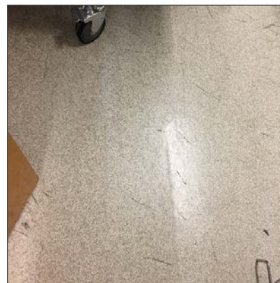
Photo 2 – Asbestos-containing vinyl sheet flooring, grey and white square pattern, First Floor Medical Storage.
