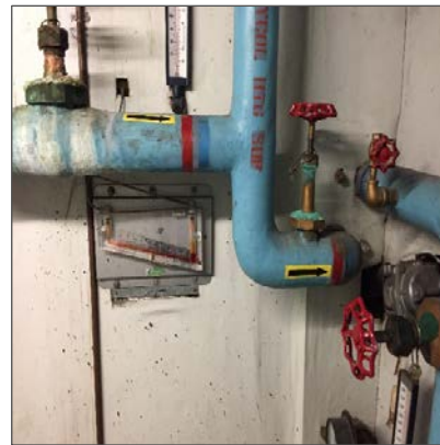
Asbestos-containing parging cement on pipe fittings, Basement Mechanical Room.
