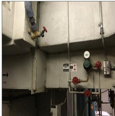
Asbestos-containing paper over fiberglass insulation – Mechanical Room #3 (sample S072A-C).
