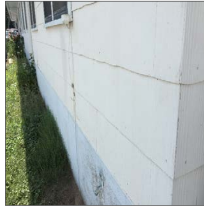
Transite exterior siding, Building Exterior.
