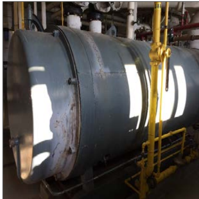
Suspect asbestos-containing insulation below metal jacketing on boiler, Basement Boiler Room.
