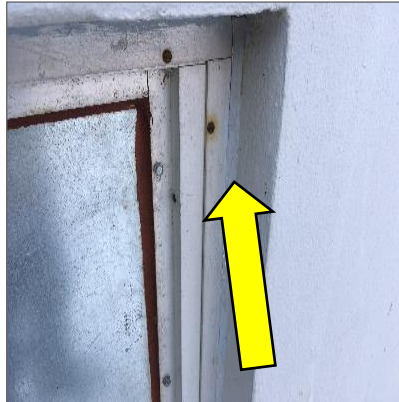
Non-asbestos grey caulking on window, Mechanical Room #1.
