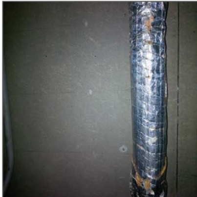
Transite board above plaster ceiling, Basement Medical Storage Room.
