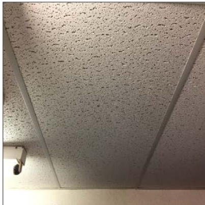
Photo 3 – Non-asbestos 24" x 48" lay-in ceiling tiles, dense pinhole and width-wise fissure, Basement Office at Sprinkler Room.
