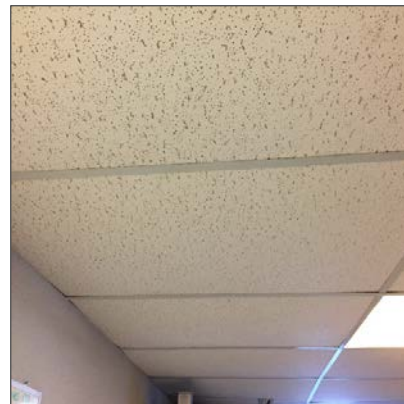
Photo 6 – Non-asbestos 24" x 48" lay-in ceiling tiles, pinhole and short width-wise fissures, Office across from Boiler Room, Basement.
