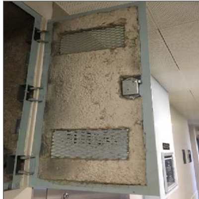
Asbestos-containing tamped firestopping in electrical panel (photo from previous assessment).
