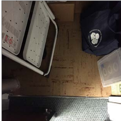
Asbestos-containing 9" x 9" vinyl floor tiles, beige with red streaks, Stationery Closet.
