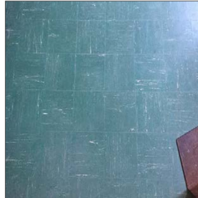
Photo 2 - Asbestos-containing 9" x 9" vinyl floor tiles, green with white streaks, Basement Inventory Storage.
