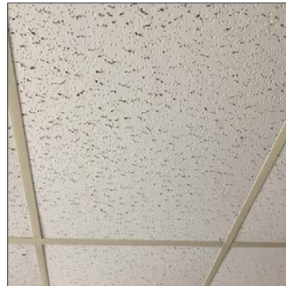
Photo 4 – Non-asbestos 24" x 24" lay-in ceiling tiles, pinhole, indent, and width-wise fissures, Basement Office.
