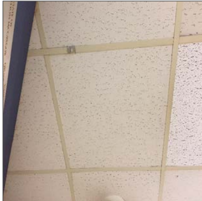
Photo 7 – Non-asbestos 24" x 24" lay-in ceiling tiles, few pinhole and width-wise fissure, Ground Floor Front Entrance.
