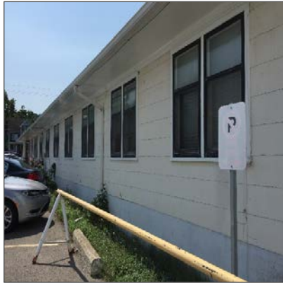
Transite exterior siding, Building Exterior.
