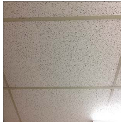
Non-asbestos 24" x 48" lay-in ceiling tiles, pinhole and small fleck pattern, Basement ECG Department.
