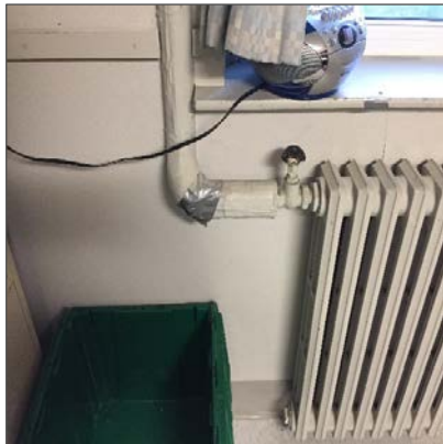
Photo 1 – Asbestos-containing parging cement on pipe fitting, fair condition, Office across from Boiler Room, Front Wing Basement.
