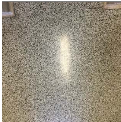
Photo 3 – Asbestos-containing mastic under non-asbestos 12" x 12" vinyl floor tiles, smaller black and white flecks, Ground Floor ER Corridor.
