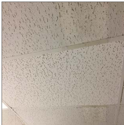
Photo 5 - 24" x 48" lay-in ceiling tile, pinhole and fewer width-wise fissure, Basement Corridor.
