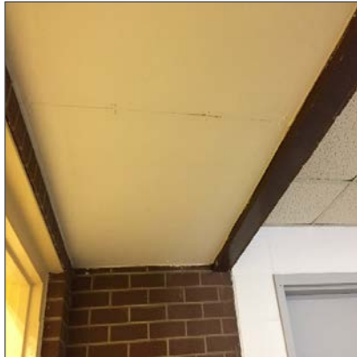
Transite board on former soffit, Basement Corridor, ER Department.
