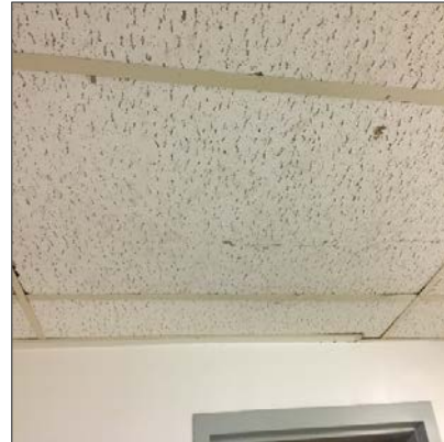
Photo 2 – Non-asbestos 24" x 48" lay-in ceiling tile, pinhole, indent, and deep width-wise fissures, Basement Corridor.
