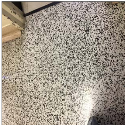
Photo 3 – Non-asbestos 12" x 12" vinyl floor tiles, larger white and black flecks, First Floor Corridor and Operating Room.
