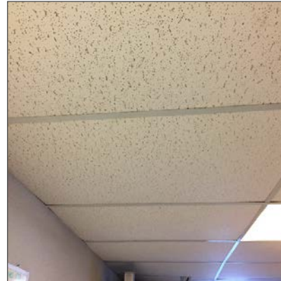
Photo 8 – Non-asbestos 24" x 48" lay-in ceiling tiles, pinhole and short width-wise fissures, Office across from Boiler Room, Basement.
