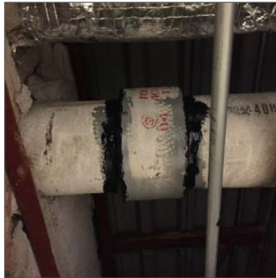
Transite rain water leader, Halfway Café Lounge.
