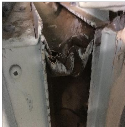
Non-asbestos textile vibration damper, Mechanical Room #1.
