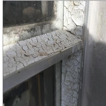
Asbestos-containing white caulking at interior windows – Boiler Room (samples S066A-C).
