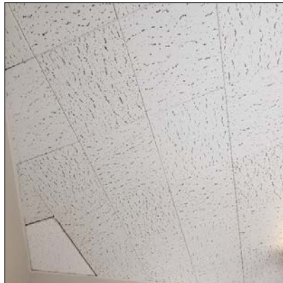
Photo 9 – Non-asbestos 12" x 12" glued-on ceiling tiles, pinhole and fissures, First Floor Corridor.
