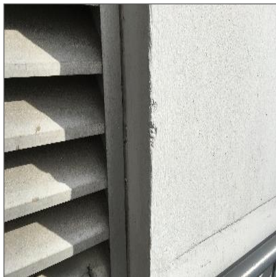
Non-asbestos grey caulking around the exterior frames of louvres – Exterior Boiler Room (samples S067A-C).
